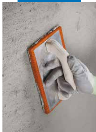
Tamping Planitop Smooth & Repair
